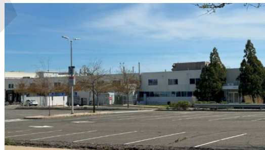
North Façade and Main Entrance of Wing G
