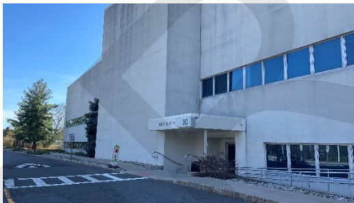
East façade of Building 30 (Wing O)
