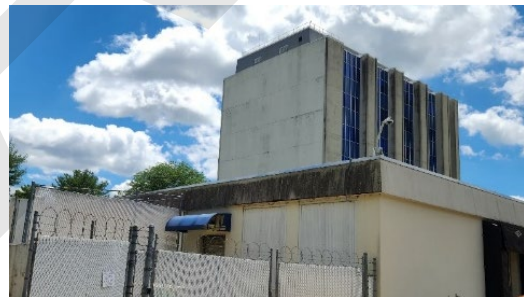
Research Tower (northwest façade)
