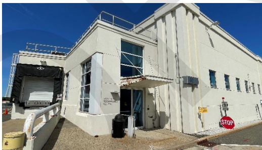
ATC entrance at southwest corner of Building 40
