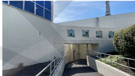
Below-grade access and structural connection between Clinic (left) and Wing G (right)
