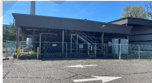
Tank Farm storage building viewed from west campus parking lot (W3).
