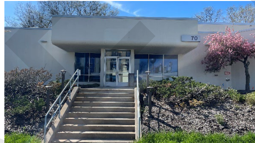
Fitness Center entrance
