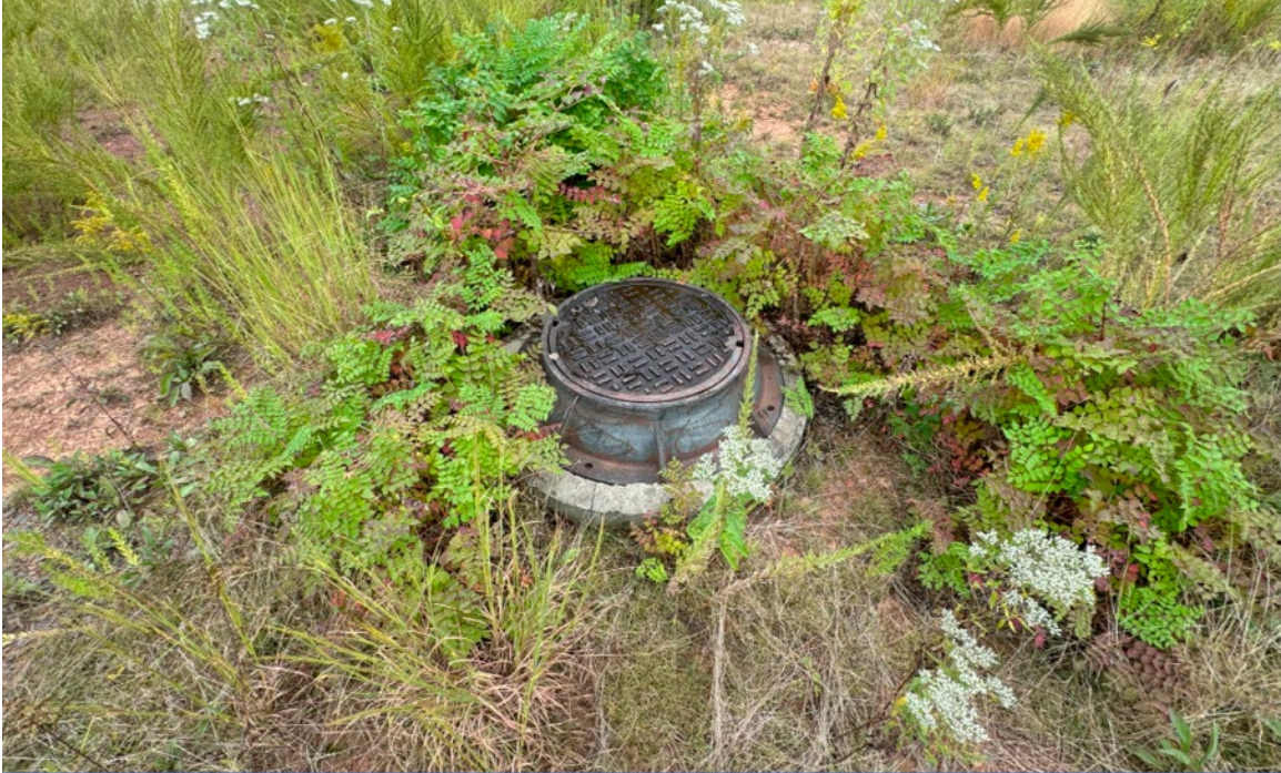
Photo 18. Existing Utility Access
