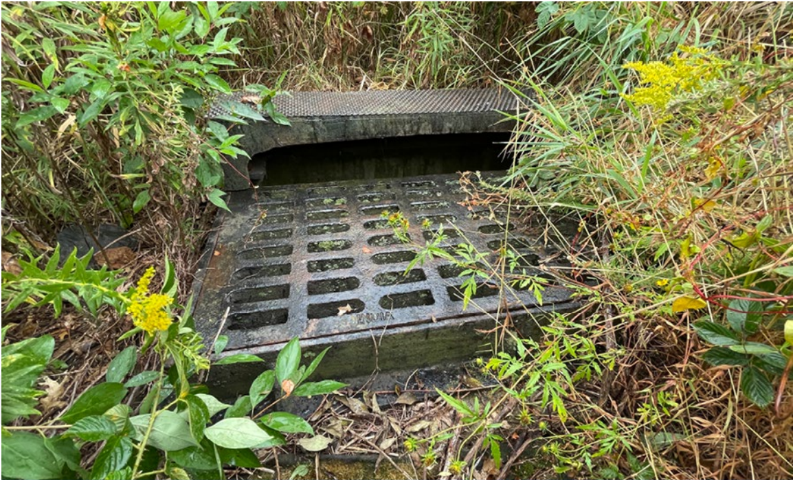
Photo 8. Stormwater Inlet At Rear Edge of Gravel Area (Lot 1.04)
