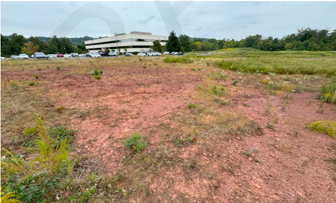
Photo 22. Exposed Soil at Building Pad (Lot 1.04)
