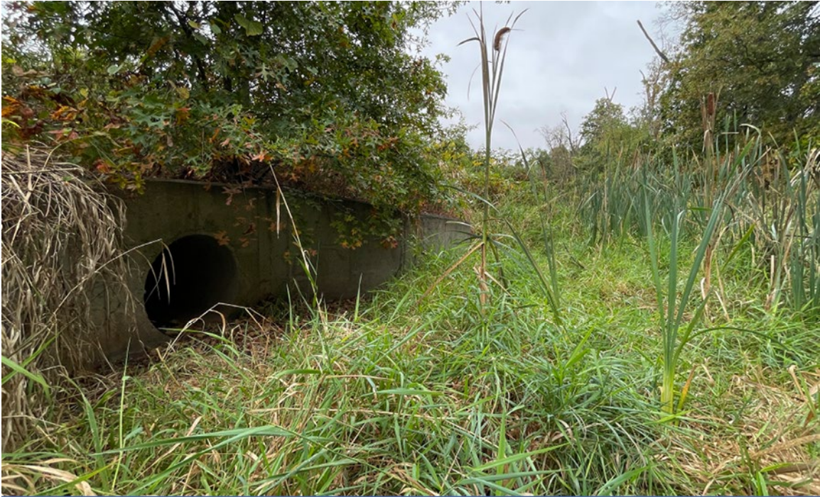
Photo 9. Headwall Outlet and Swale (Lot 1.04)
