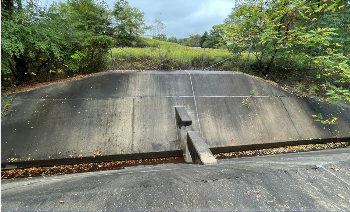
Photo 11. Concrete Spillway and Outlet Control Structure (Lot 1.02)
