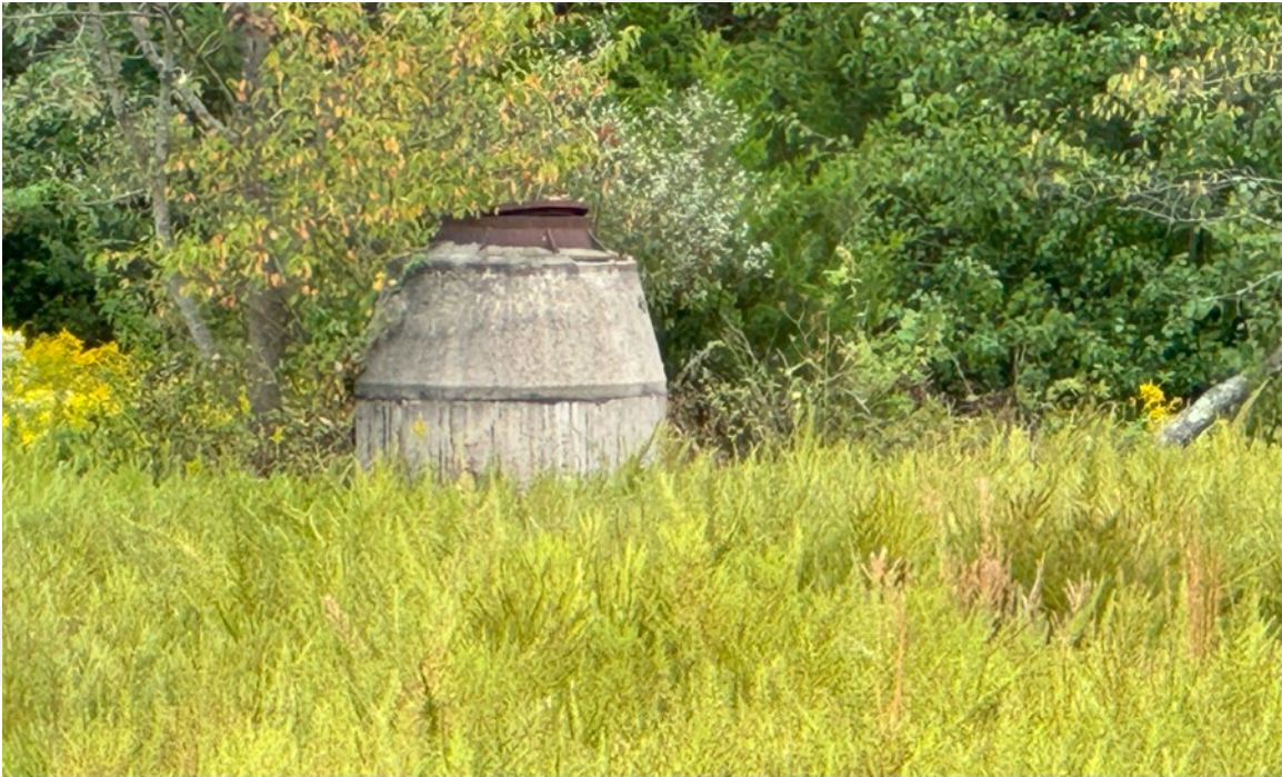
Photo 24. Existing Sanitary Sewer Manhole (Lot 1.02)
